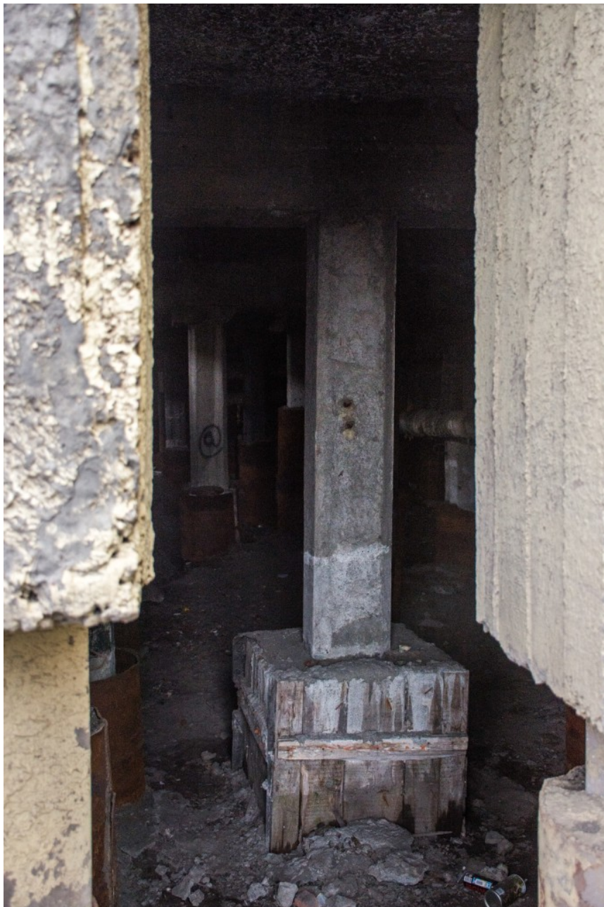
Peering into the lifted foundation of a building in Norilsk (Credit: Olga Dobrovidova)
